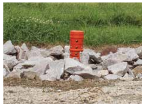
A drain tile surface inlet to remove ponded water from fields quickly.
